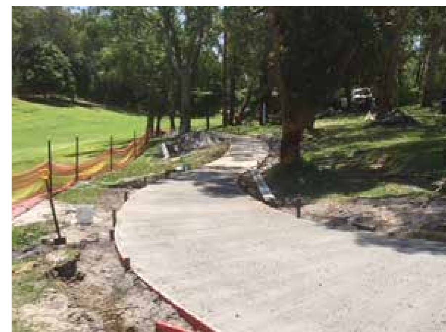
THE NEW PATHWAY ALONG THE 19TH FAIRWAY HAS BEEN COMPLETED
