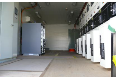
Simberi Gold Equipment Installed
