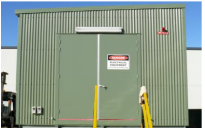
Dunheved Pumping Station 1501
