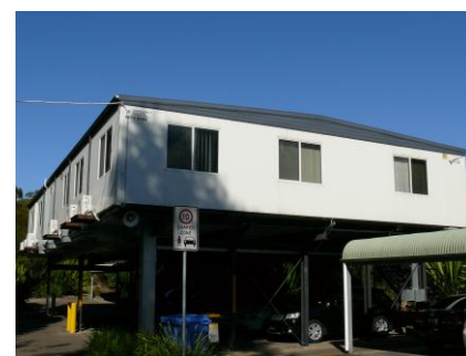
Parking Gantry Level
